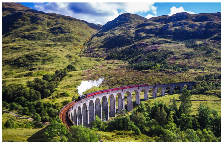
Journey aboard the West Highland Line across the iconic Glenfinnan Viaduct.
